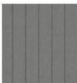
2. Vertical standing seam zinc cladding - adhering to the language of a mansard roof
